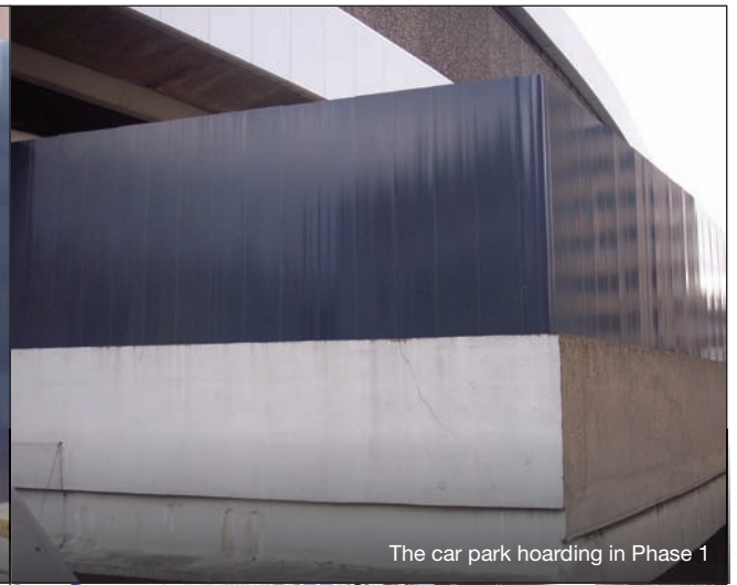
Temporary gates allow access in Phase 1
