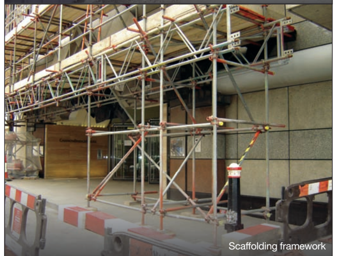
Cup lock and standard scaffolding
