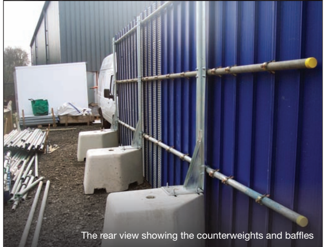
Kings Cross, counterbalanced support system
